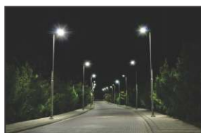
Solar Street Lighting
